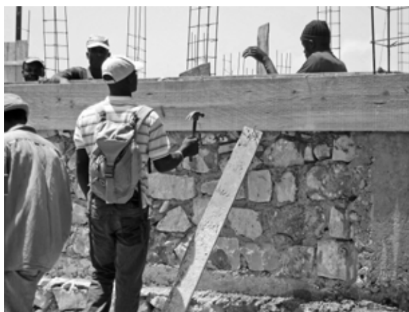
Ongoing construction at Dumas A rocks made 4 rooms building.
