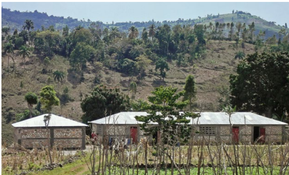
The Clermont school, which I visited end of 2014, was extended (see above on the left). The second building with three classrooms at Philo (picture in the 114 issue) was completed in February.
